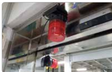
▶ Inside&Outside Office at Factory / Flashlight ZT
